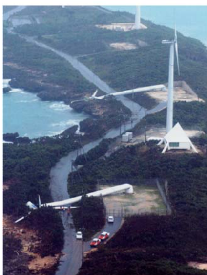
Fig. 1 Damaged wind turbines on Miyakojima Island during Typhoon Maemi in 2003
