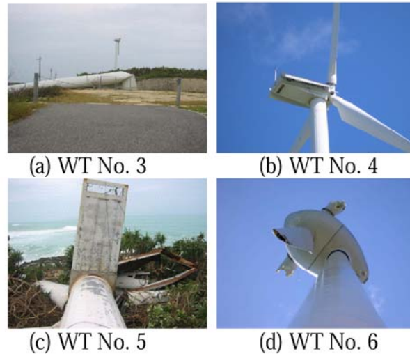
Fig. 7 Damaged wind turbines at Karimata
