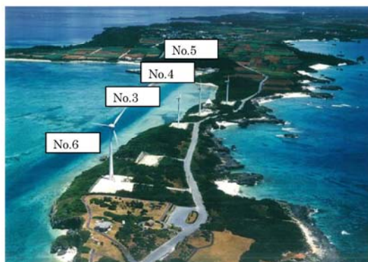
Fig. 6 Turbines at Karimata before the damage
