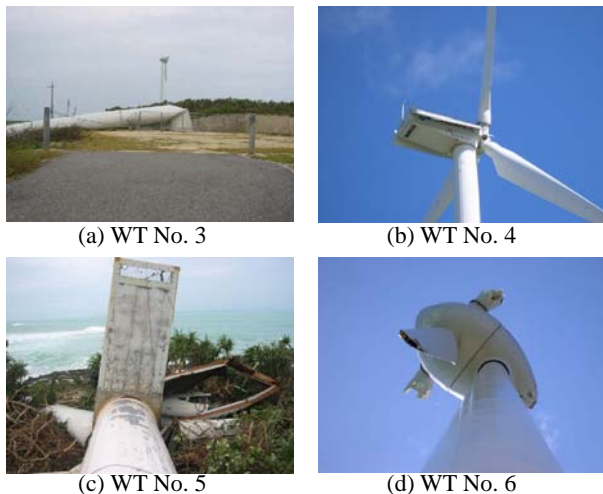
Fig. 7 Damaged wind turbines at Karimata
