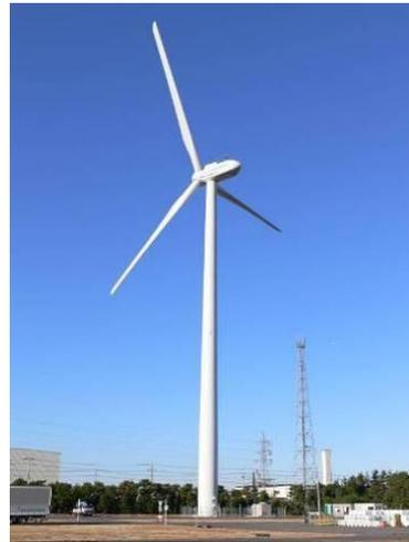
Figure 1 HTW2.0-80 downwind turbine<sup>3</sup>
