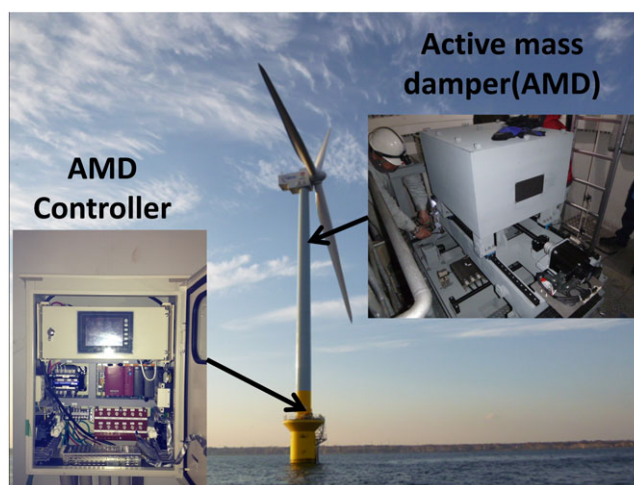
FIGURE 3 Outline of the target wind turbine and the active mass damper [Colour figure can be viewed at wileyonlinelibrary.com ]
