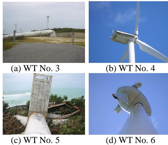
Fig. 7 Damaged wind turbines at Karimata
