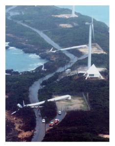
Fig. 1 Damaged wind turbines on Miyakojima Island during Typhoon Maemi in 2003
