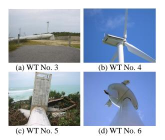
Fig. 7 Damaged wind turbines at Karimata
