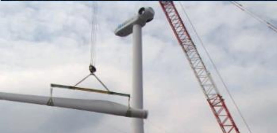
The 2MW downwind offshore wind turbine was installed in June, 2013. At first the 48.5m tower divided into three sections and the nacelle were assembled and then 39m blades were installed. Commissioning test was carried out after towing to Onahama port.
