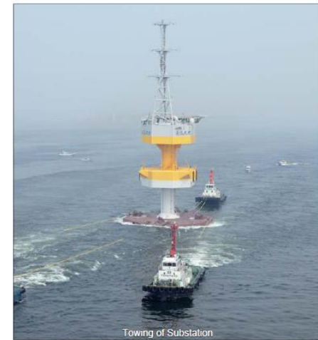
Towing of Substation
