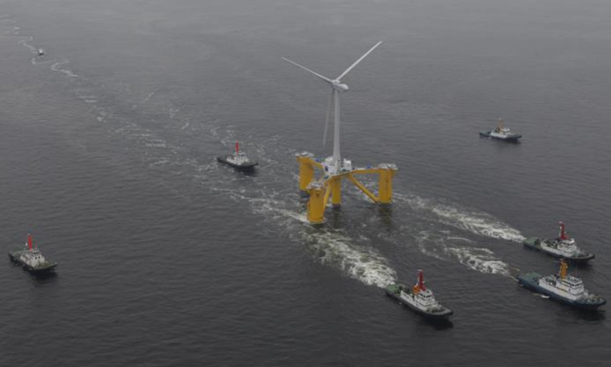
This huge floater was towed from Chiba to Onahama and then to the installation site, offshore 20km of Fukushima. Three front tugboats and one rear boat were used. There were four boats for towing in total.
