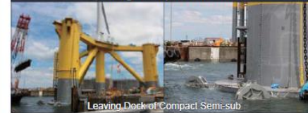
Leaving Dock of Compact Semi-sub
