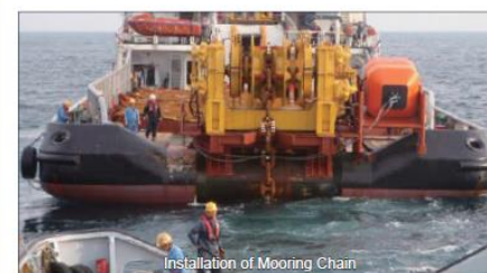
Installation of Mooring Chain
