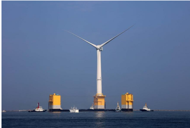
MHI's 7MW floating turbine has been installed off Fukushima
