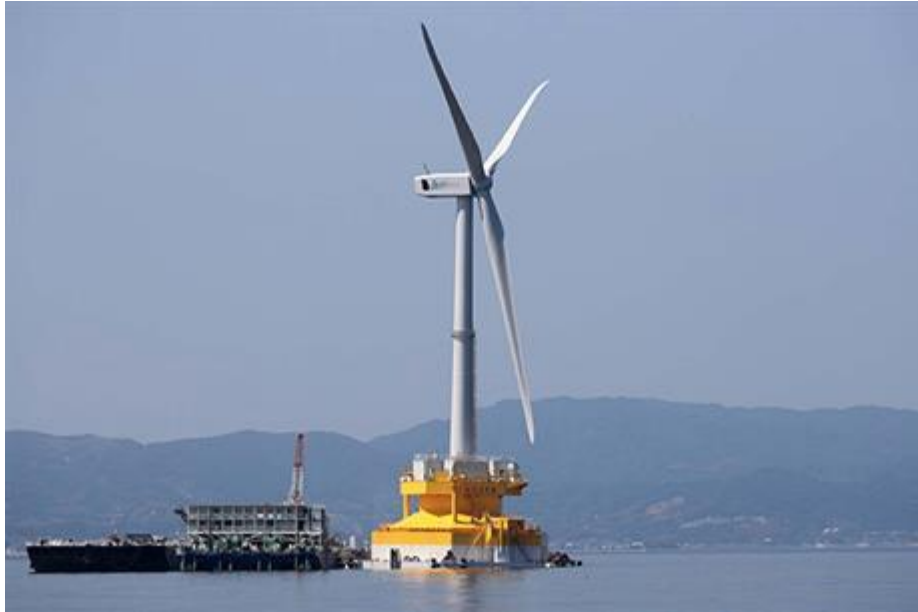
A prototype of Hitachi's downwind 5MW turbine is being installed in Fukushima, Japan
