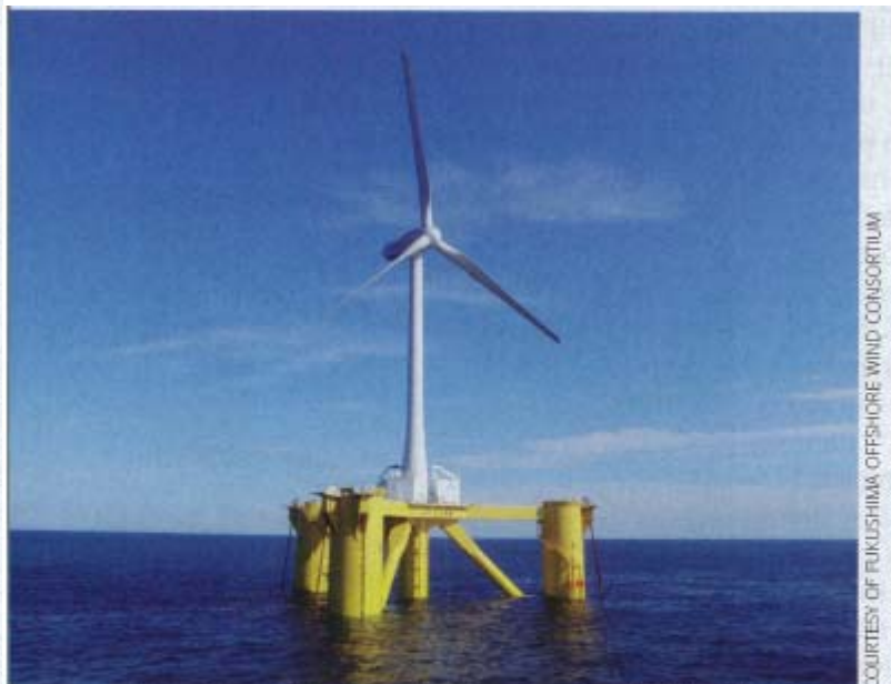
Fukushima Mirai, a wind generation facility floating about 20 kilometers offshore of Fukushima Prefecture
