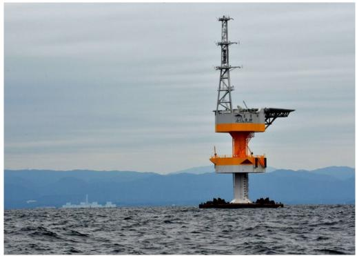
Yoshikazu Tsuno/Agence France-Presse — Getty Images The project's turbines, and even the substation and electrical transformer equipment, float on giant platforms anchored to the seabed.
