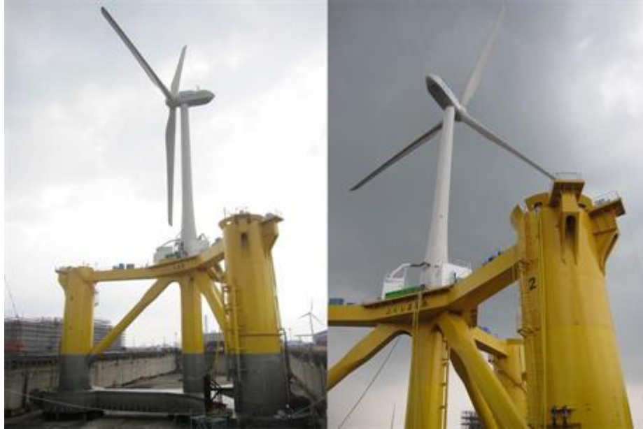
A 2MW turbine to be floated 20km off Fukushima
